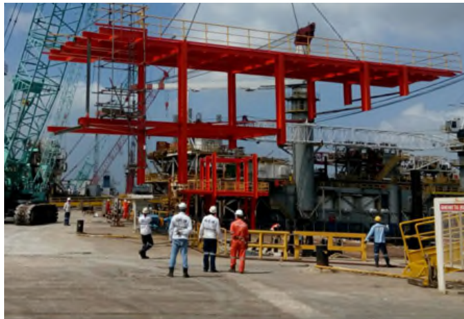
Loading Turret Trolley Support Structure
