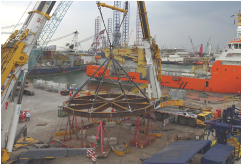
Load Testing for Turret Main Bearing Lifting Frame
