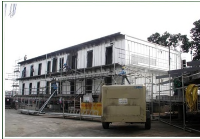
New Construction of Living Quarter Module
